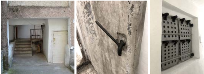
Fig. 9 (a) Entering the shelters of the basement of buildings, (b) reinforced door, (c) the element of closing window in case of bombing
