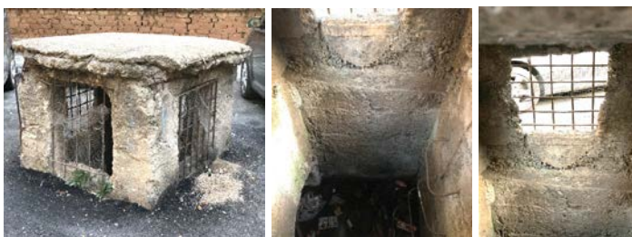
Fig. 11. Air Exchanger positioned in the courtyard that also served as an emergency exit
