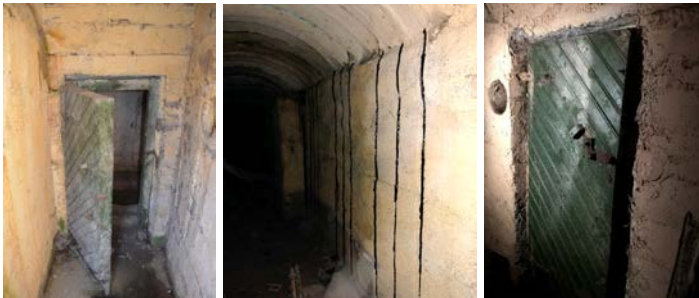
Fig. 14. (a) Entrance, (b) internal spaces, (c) openings for ventilation
